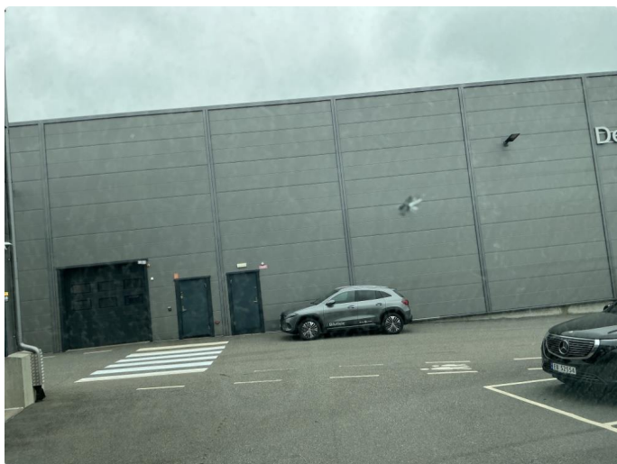
1.2 Steinsprut i synsfelt
