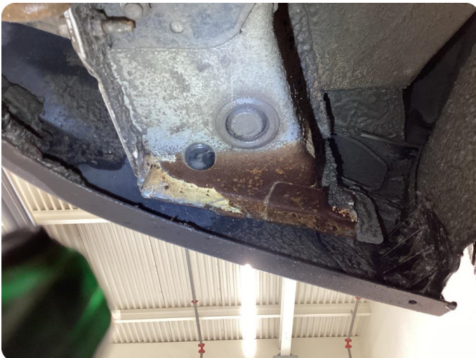
1.2 Rust Anbefaler rust behandling under
